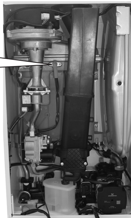
Flame Detection Electrode
