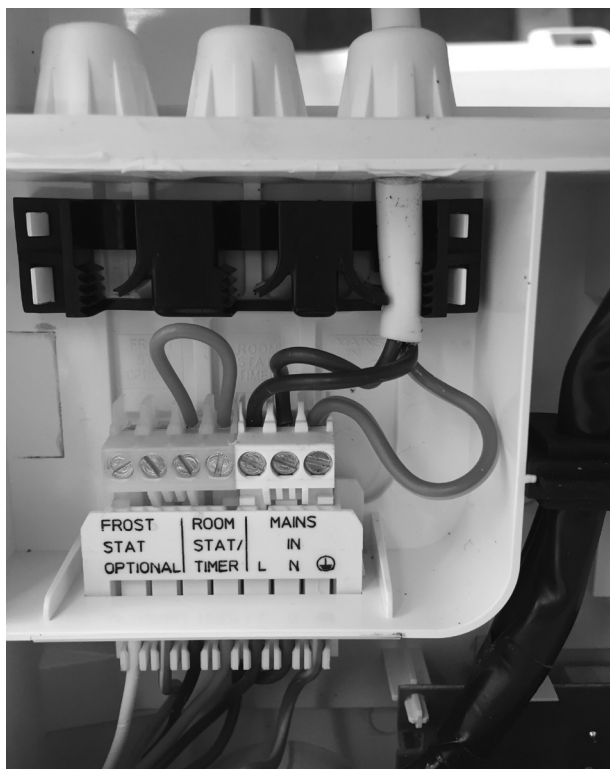
INSTALLER CONNECTIONS (LHS)
